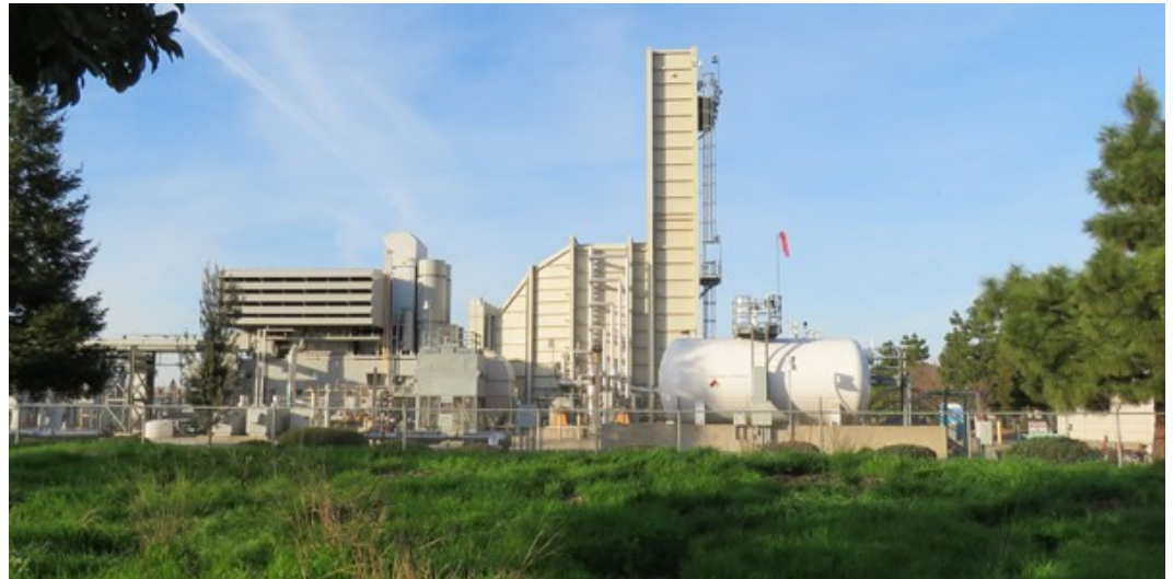
Economic pressure on natural gas plants in CAISO has led to reliability payments for Calpine's Yuba City Energy Center. | © RTO Insider
